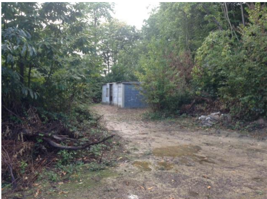
Photo 2 – Cleared Area to the South of the Roadway Showing Structure
